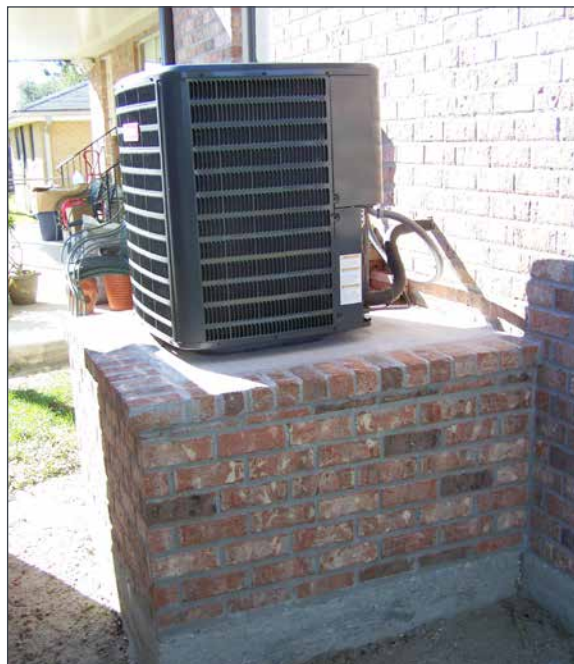
Elevated exterior HVAC equipment
