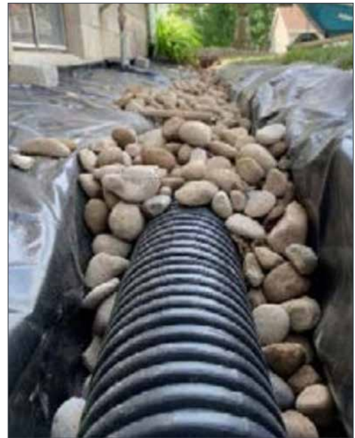
French drain around basement
