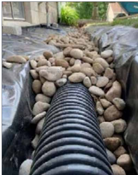
French drain around basement
