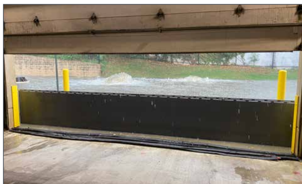
Passive flood gate at entrance to parking garage
