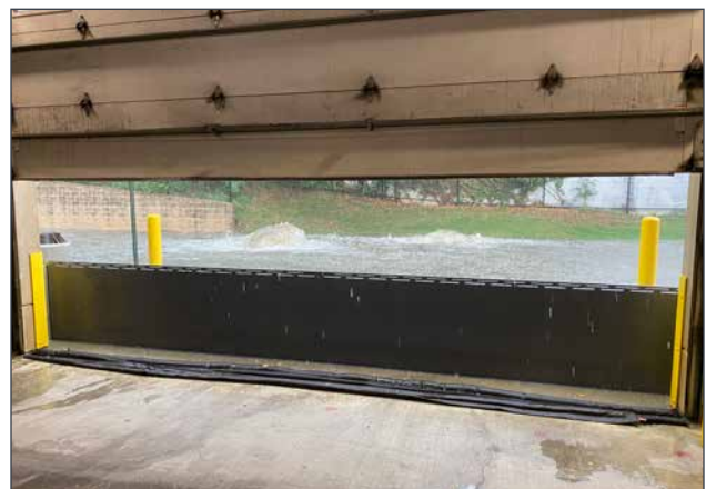
Passive flood gate at entrance to parking garage
