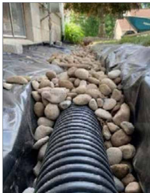
French drain around basement
