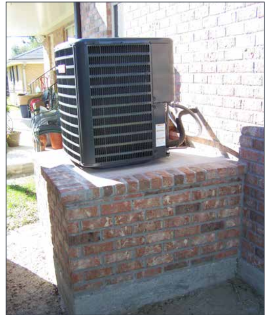
Elevated exterior HVAC equipment
